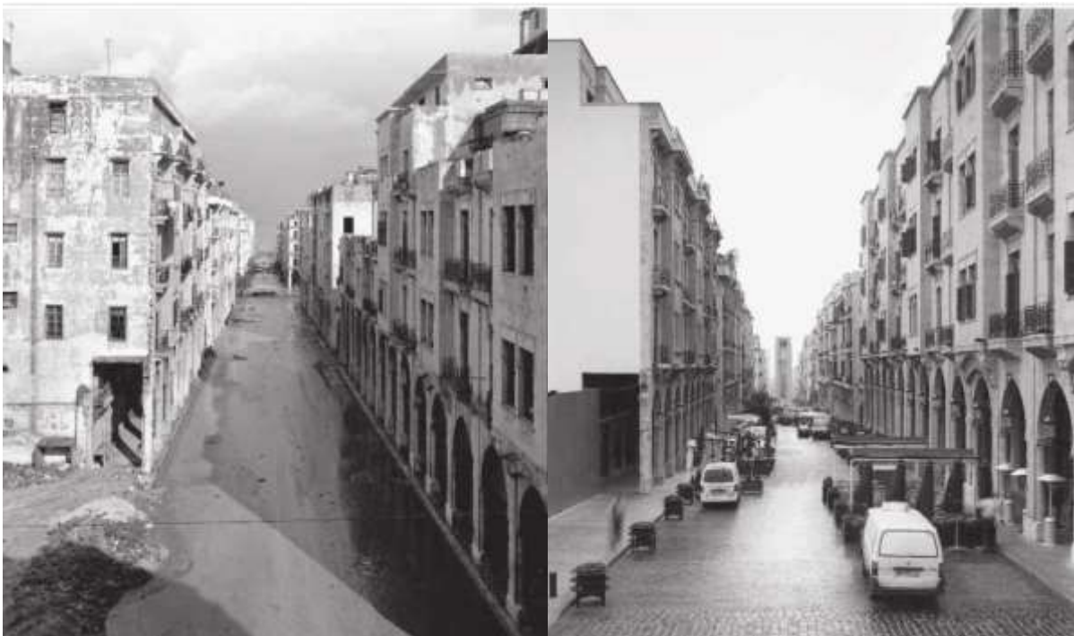
Fig.6: One of Beirut's downtown streets in 1991, and then after the conservation process in 2003. Reference: (Solidere, 2010)
